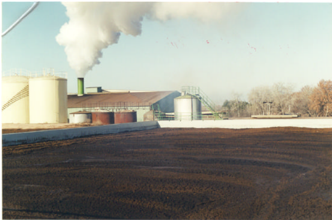
Dry spent olives installation
