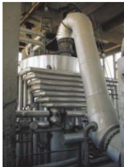
Installation of a new toaster unit
