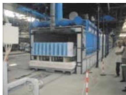
Installation of a new sanitary furnace that runs on natural gas
