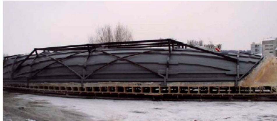
Figure 1.2. Mould reinforced with steel
