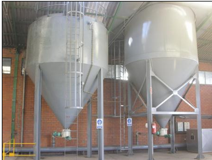
Image 7.2: Storage of petroleum coke in silos
