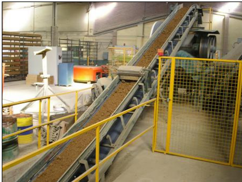
Image 3.2: Transportation of clay within an installation using rubber belts
