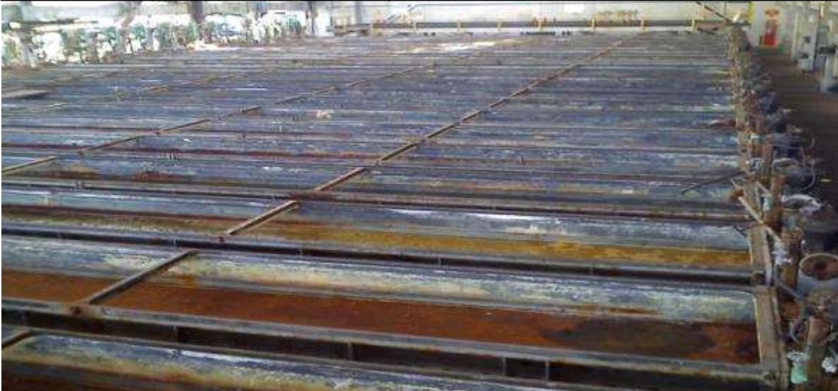
End of first dismantling stage
