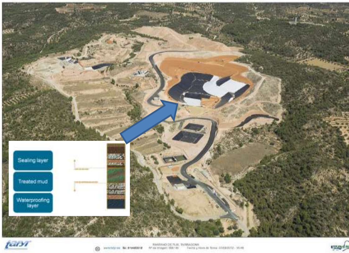
Conditioning works in the “Racó de la Pubilla” Landfill
