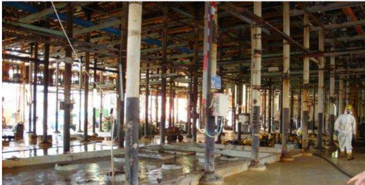
Floor of cell room regularly washed down
