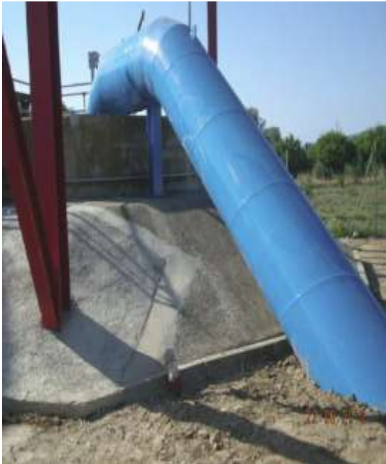
One of the wells constructed for drinking water supply to downstream towns in case of emergency
