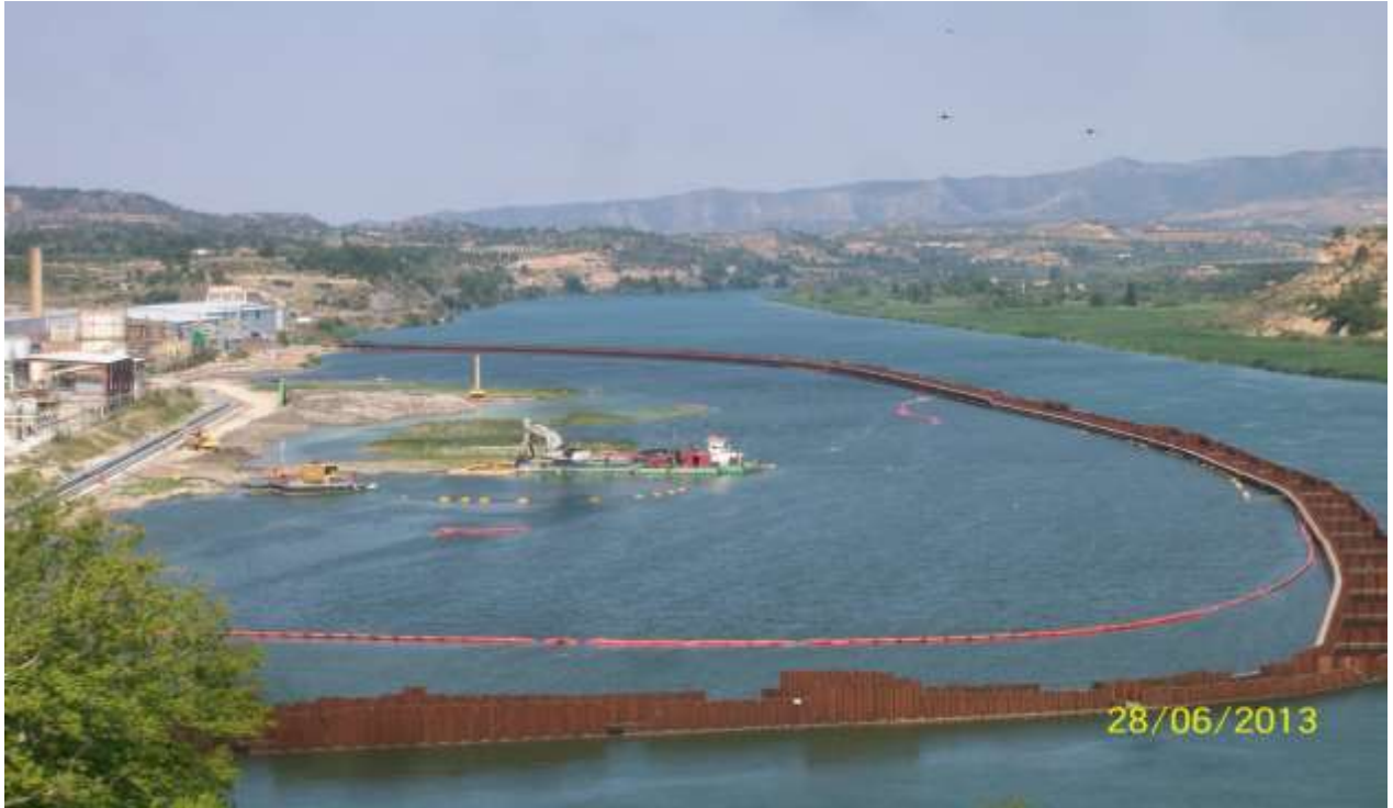
Dredging activities inside the sheet piling
