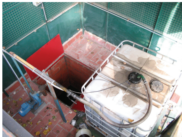
Photograph 8 CUTTING OIL GRAVITY COLLECTOR
