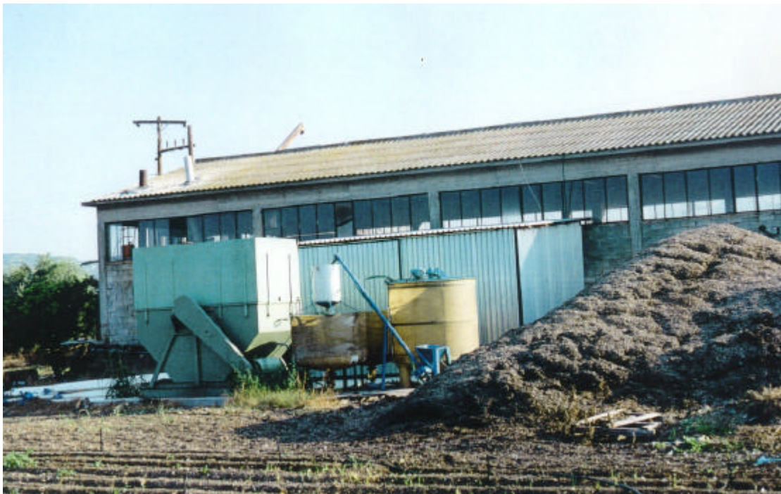
Pilot plant for the transformation of vegetable water into liquid fertiliser in Romanos, Messina (Greece)
