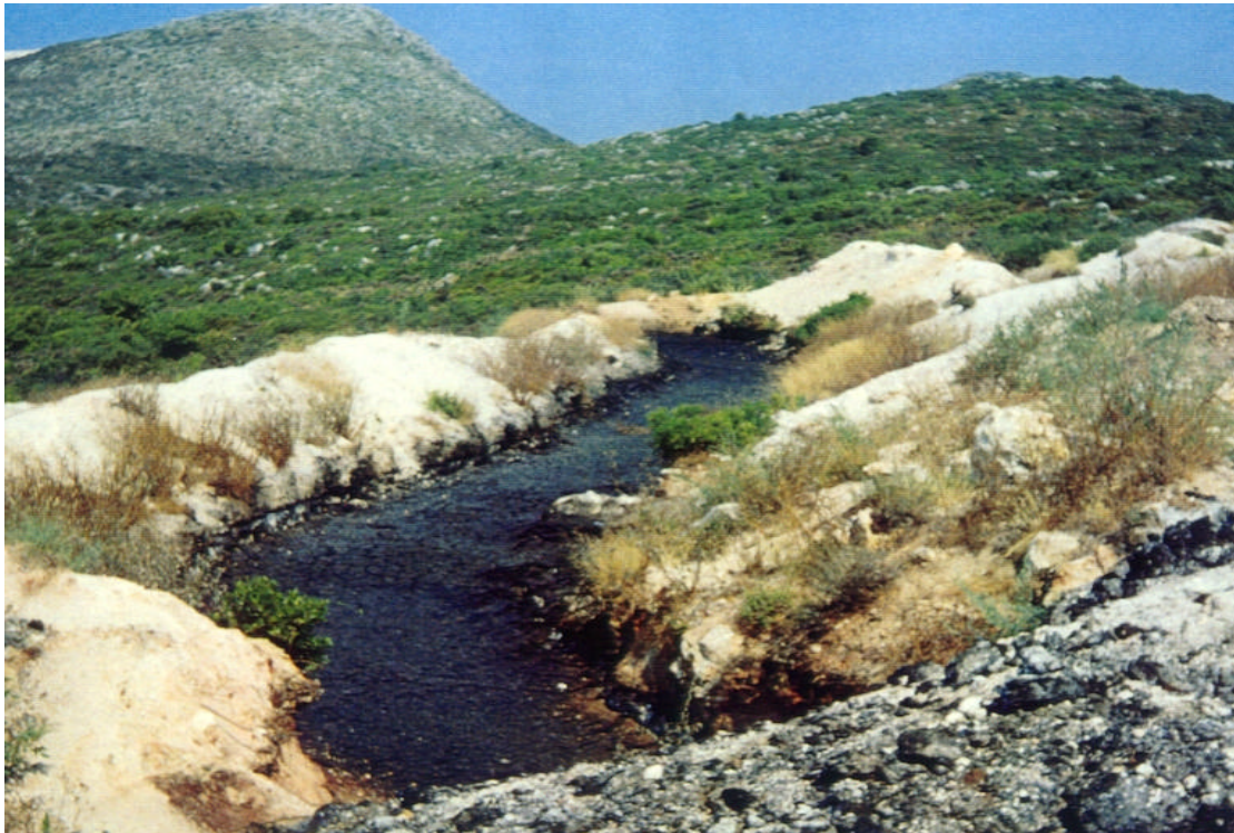
Reservoir system used in Greece to storage/evaporate vegetable water
