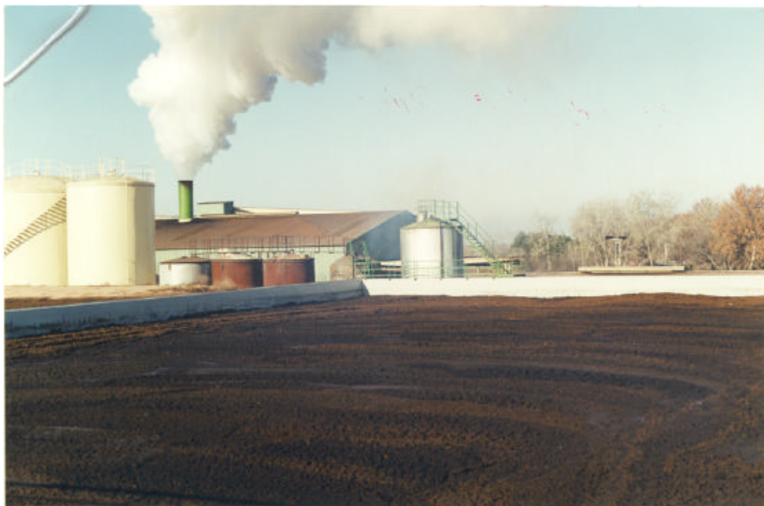
Dry spent olives installation
