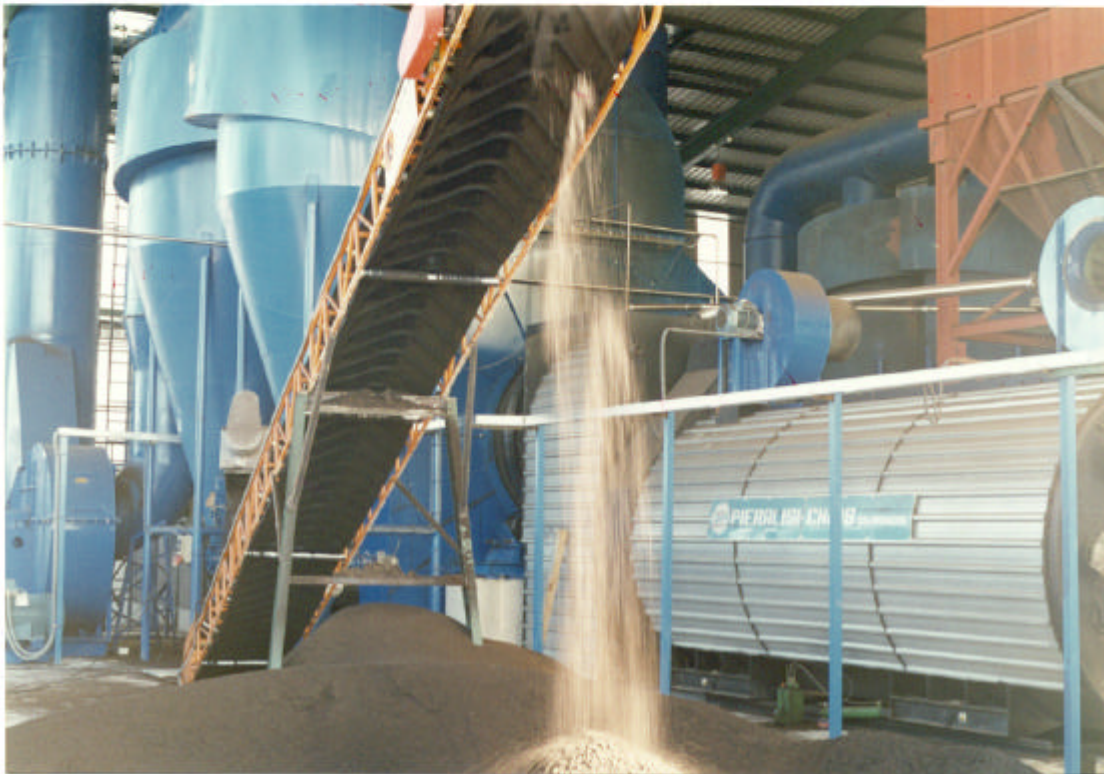
La Gineta plant (Albacete) – Dryers
