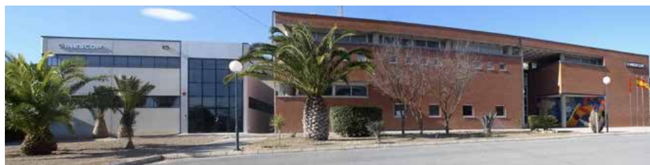
Figure 1. INESCOP's Headquarters in Spain
